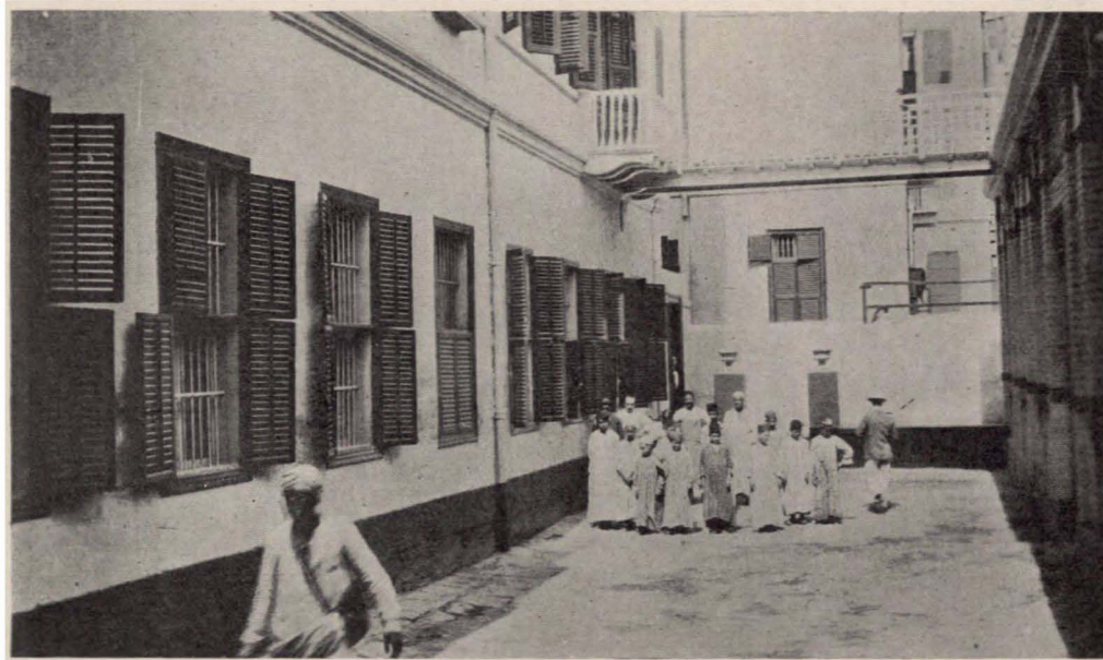
LOWER PART OF MAIN BUILDING, SHEWING LITTLE BRIDGE ACROSS FROM SUPERINTENDENT'S ROOM TO ROOF OF MACHINE ROOM, WITH GROUP OF BINDERS.
